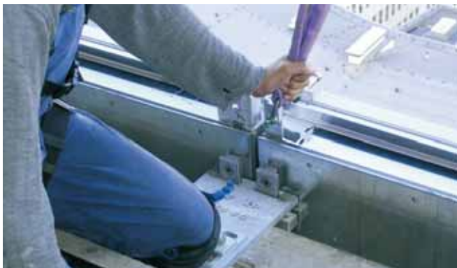
Fixing of a modular façade using HCW-ED Brackets on HTA-CE Channels
