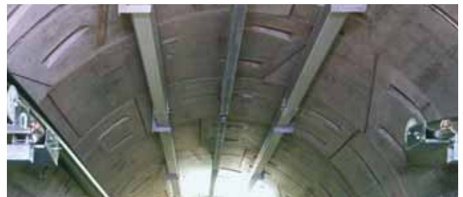
Curved HALFEN Cast-in channels in tunnel segments
