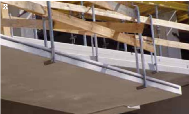
①-④: Safety rail installation, multi purpose arena in Berlin
