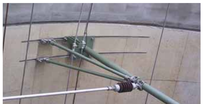
Fixing of overhead cables in railway tunnels
