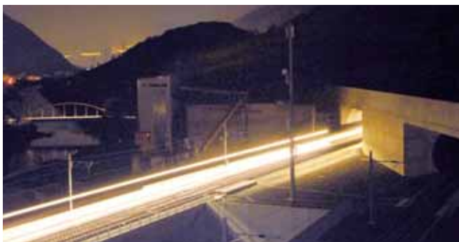
Lötschberg-Base tunnel, Switzerland
