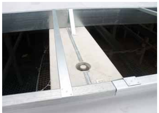
HALFEN HTU Cast-in channels in a pre-stressed concrete beam
