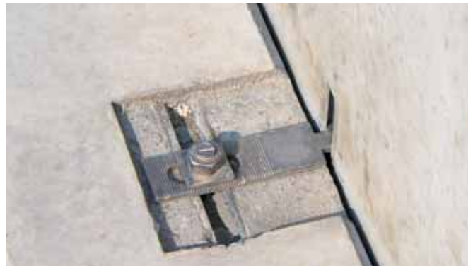
HALFEN HKZ Restraint tie with serrated washer
