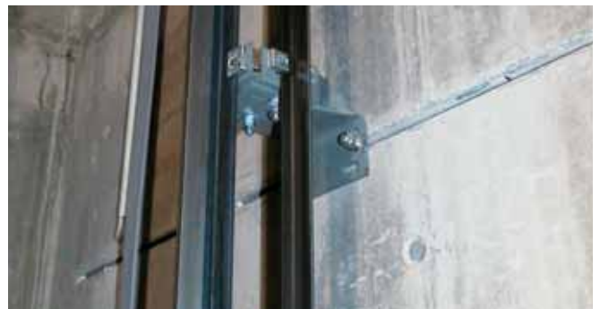
Fixing guide rails with HALFEN Channels
