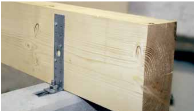
Connecting construction timbers to concrete using the HNA
