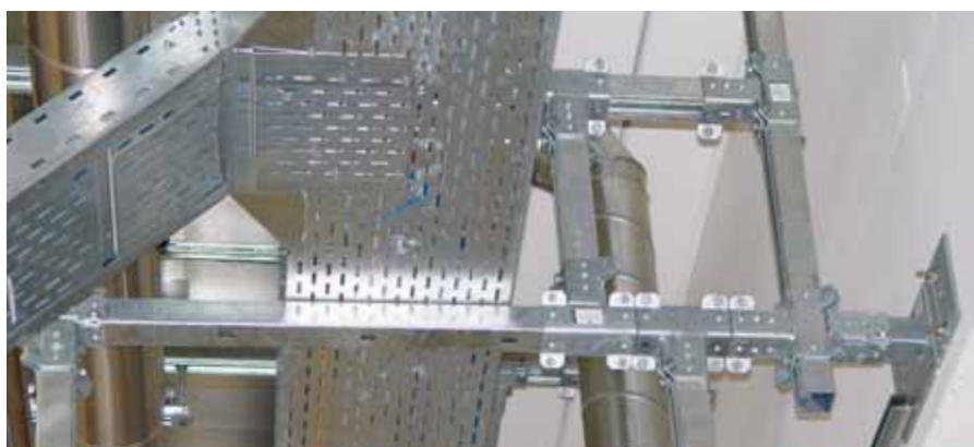
Typical application of the HALFEN Powerclick system
