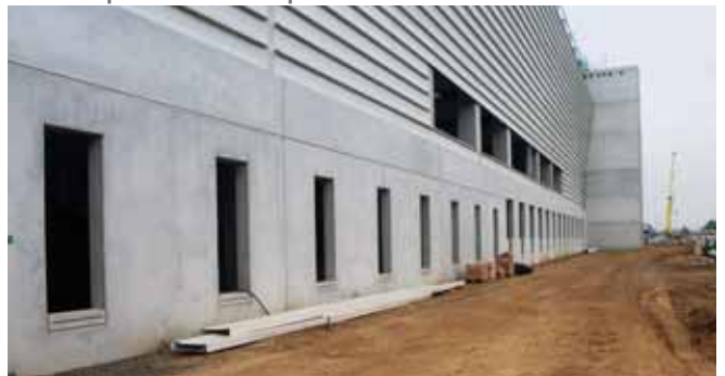
UPS Air Hub, Cologne Bonn Airport, Germany
