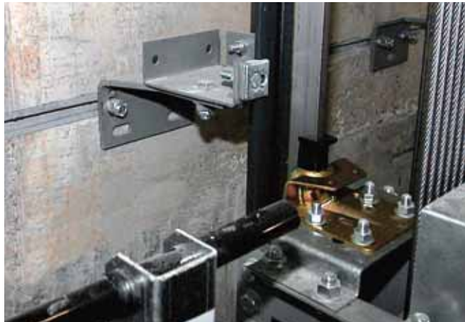
Fixing for guide rails
