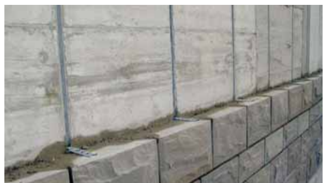
HALFEN ML Brick-ties anchor system
